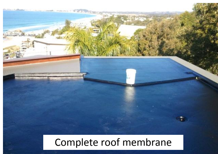
Potable seamless membrane complete
